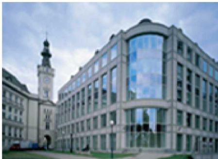
BRE Bank SA, Poland • Architects : Bielyszew, Czyz, Kleinert
