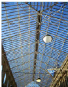
Glass roof, St Nicholas Market, Bristol
