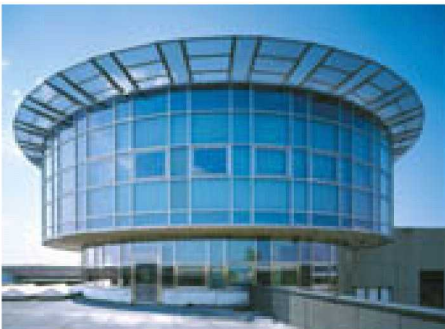
Fergamma Offices, Italy Architect : Amerigo Berto
